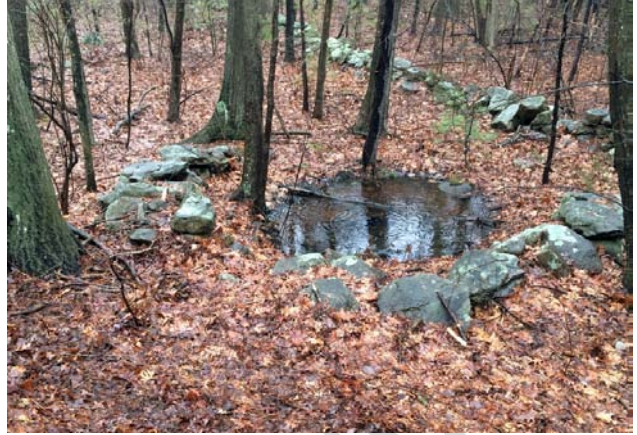
This water hole at Franklin State Forest is believed to have been constructed by the CCC. The stone wall visible in the foreground and on the left side of this photo once encircled the entire water hole. (See Appendix K for photo information.)
