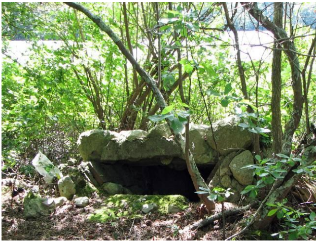
A collapsed chimney near the junction of Hawksnest and Black ponds marks the former location of a duck hunting camp. (See Appendix G for photo information.)
