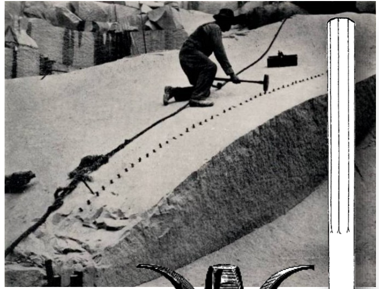
A quarry worker used a hand drill ( far right ) to make holes in the stone for explosives, or to split the stone using plugs and feathers ( near right ), as seen above.
