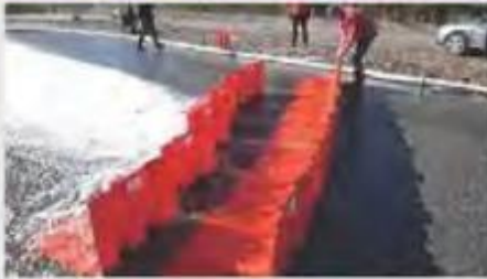
Photo courtesy of NOAA BOXWALL FLOOD BARRIER
