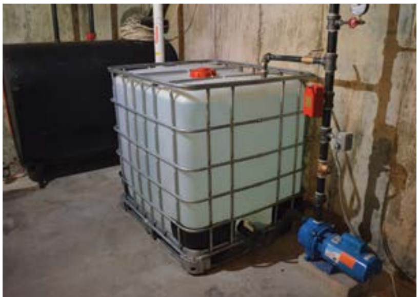
The installed sprinkler system water tank. The collapsible plastic tank has a metal frame that holds the weight of the water.
