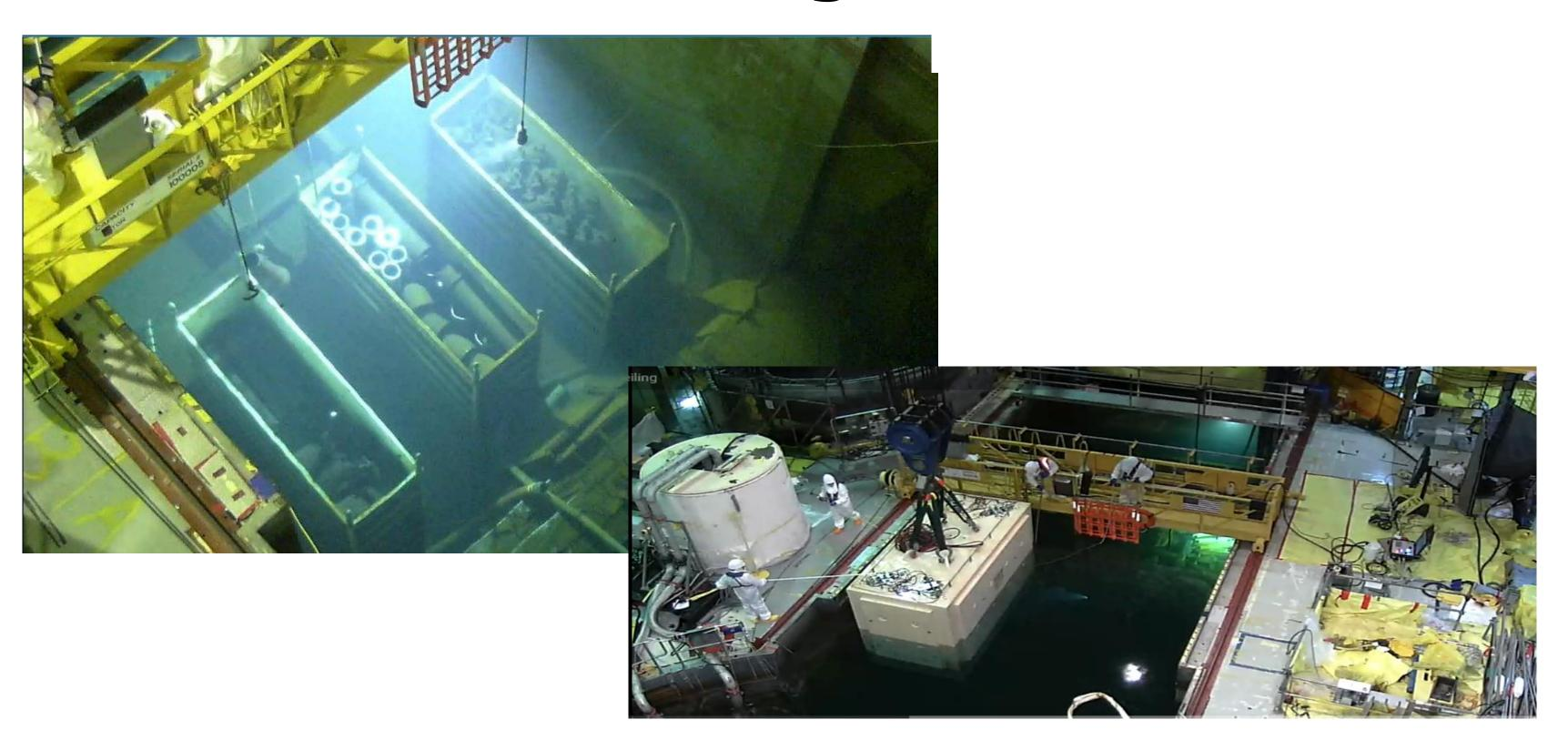
Vessel Internals Segmentation Complete Removal of equipment from DSP and Cavity In Progress
