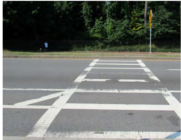
Right: The crosswalk across Morton Street at the MBTA bus stop looking south. Note the lack of wheelchair ramps at entering the crosswalk and at the Morton Street median.
