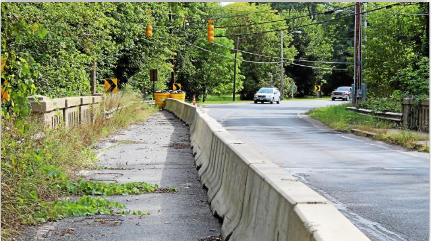
Route 7 bridge, north of Sheffield Center Source: Berkshire Eagle
