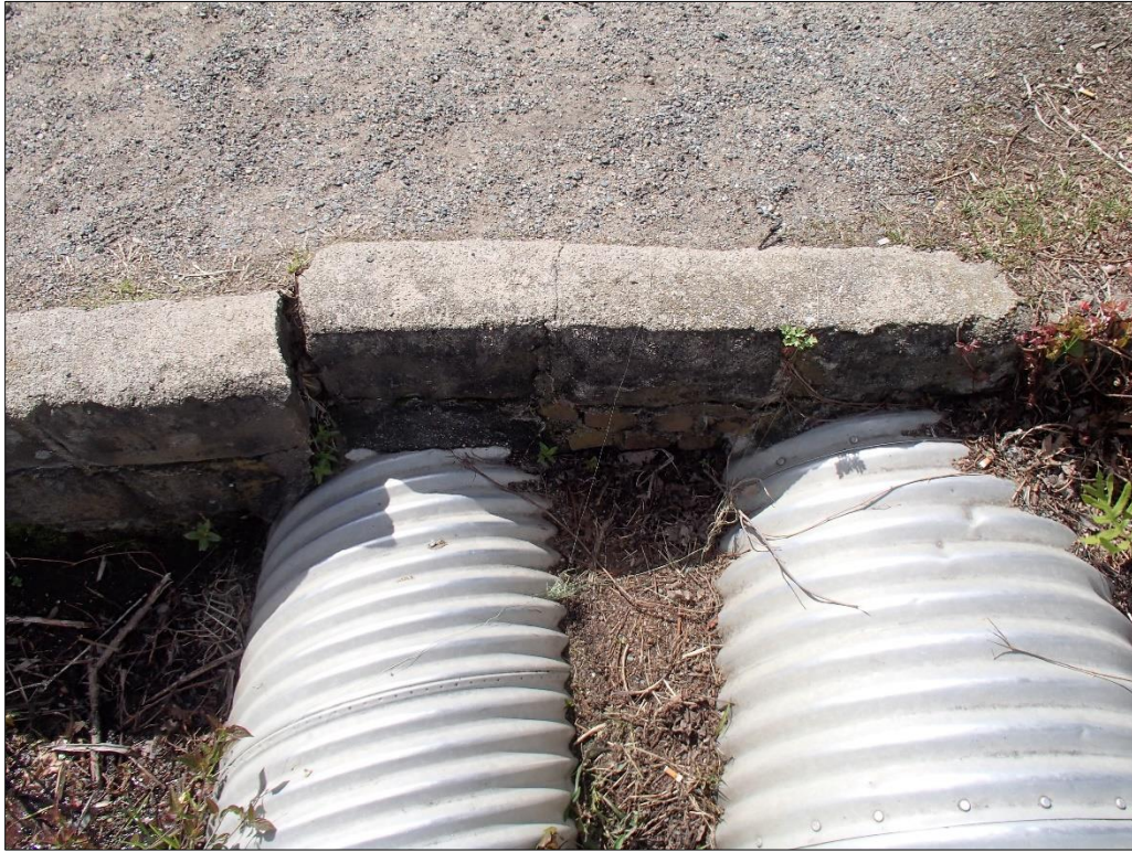
Photo 5 Looking South: North Headwall at CMPs
