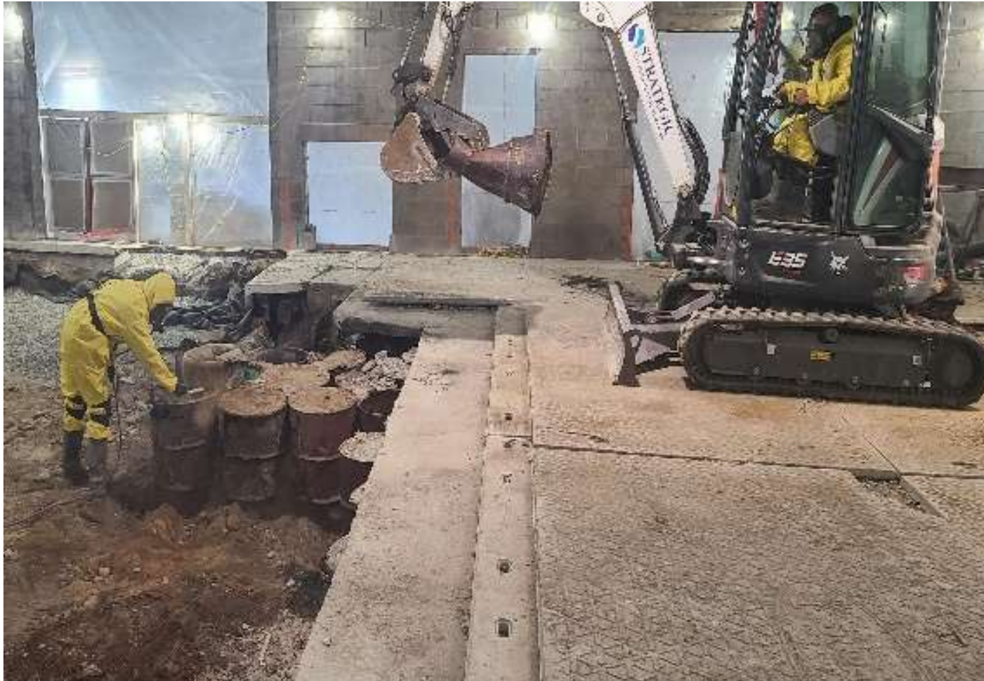
Removal of drums found inside a building under a concrete floor during redevelopment of the property.
