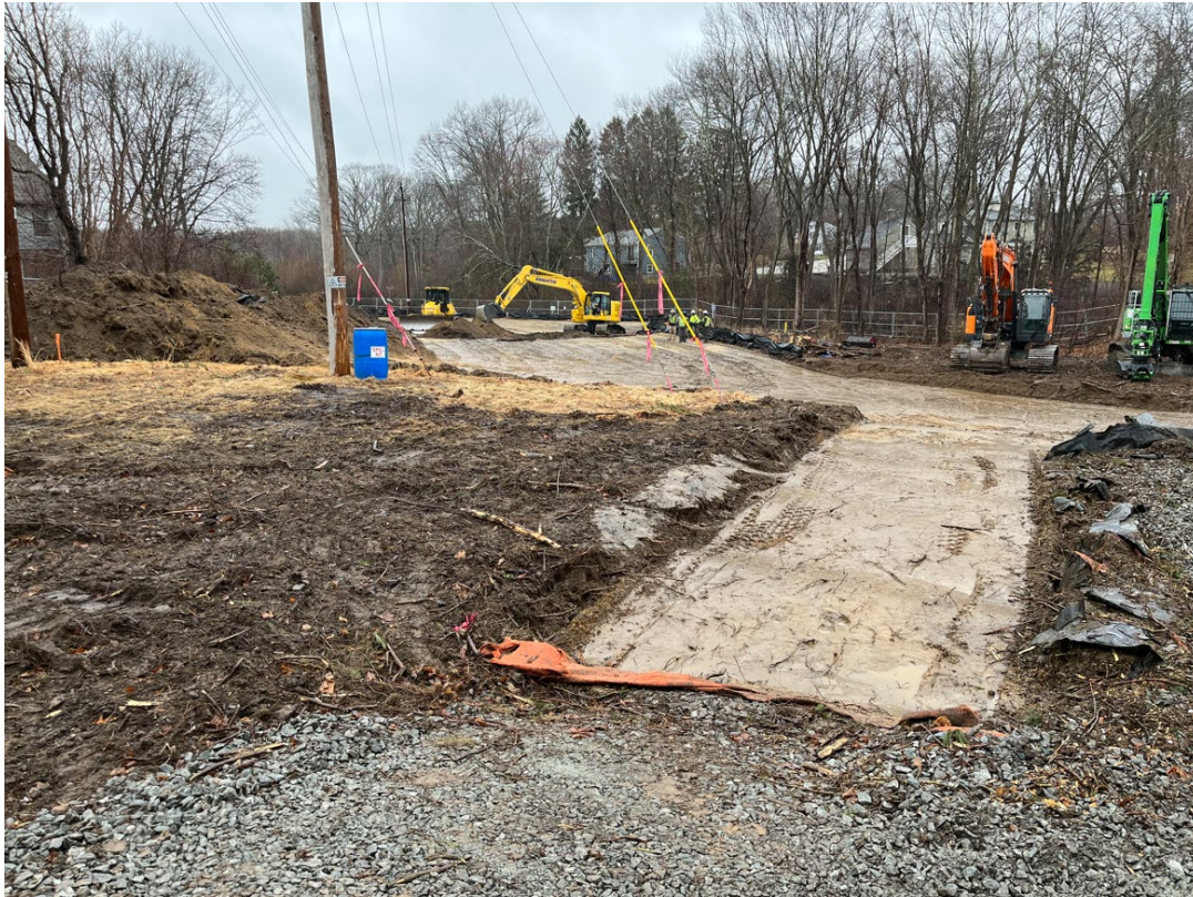
Platform Construction in preparation for Permeable Reactive Barrier Installation
