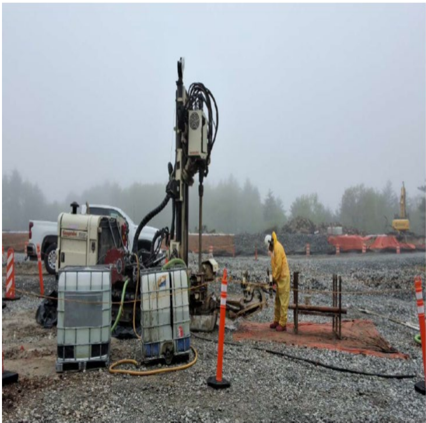
In-Situ Sequestration (ISS) in former Holding Basin
