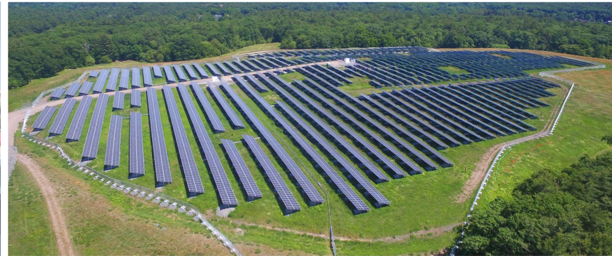
Solar on capped landfill - Beverly
