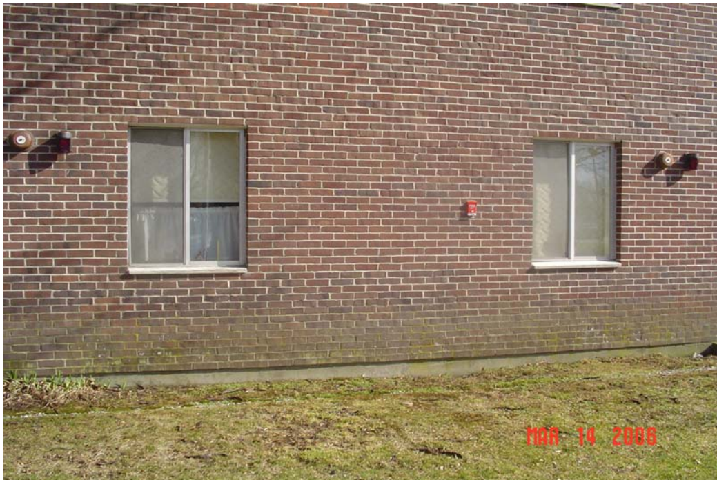
667-1 Development, John F. Kennedy Terrace Building 5 Exterior – Brick Siding in Need of Repointing
