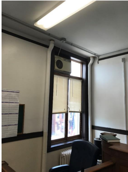
Photo 1 - Typical Window With AC Unit
