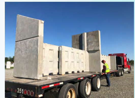
Precast Culvert Delivery
