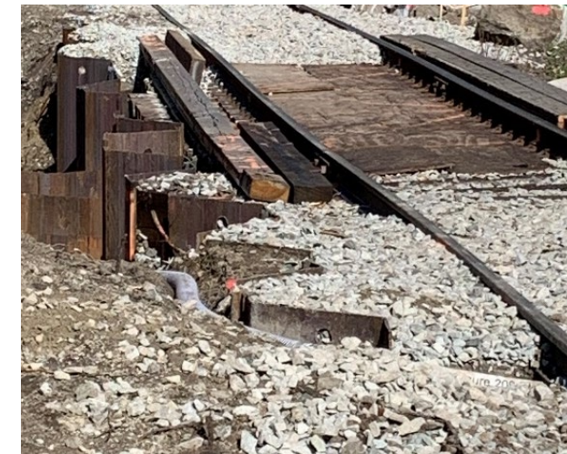
Cofferdam Installation
