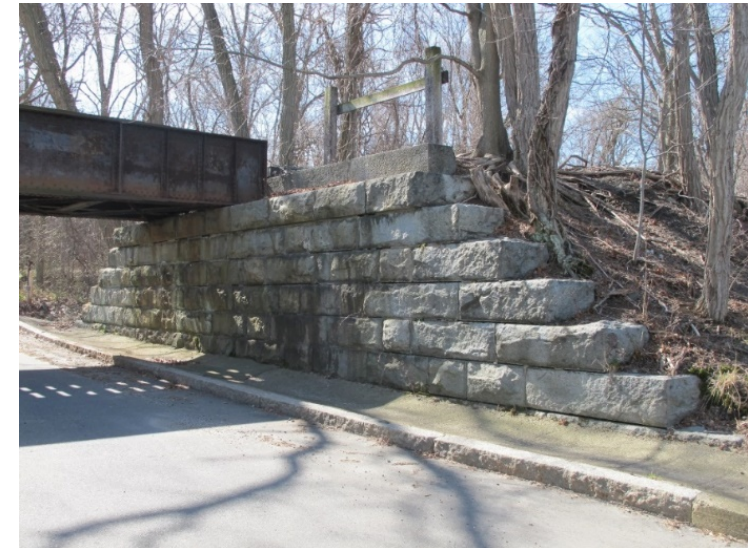
Collins Street, South Abutment and Drainage Trough
