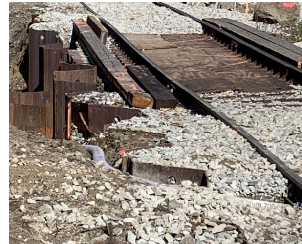
Cofferdam Installation
