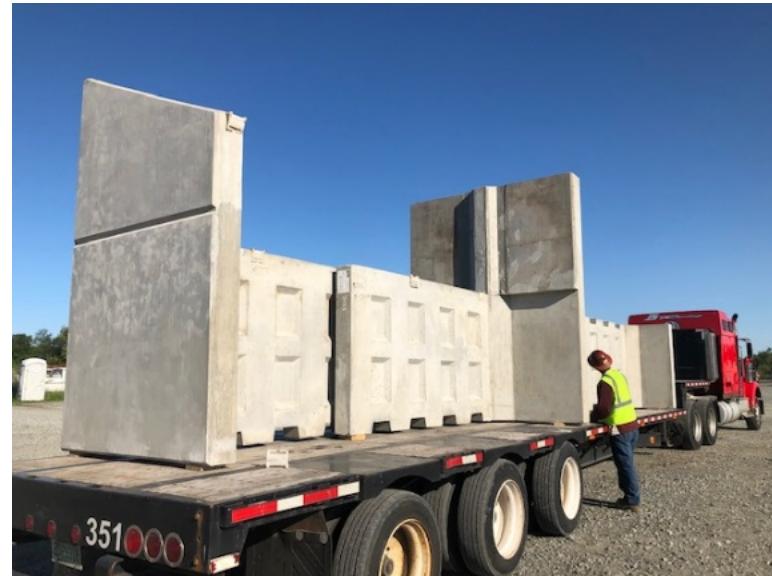
Precast Culvert Delivery
