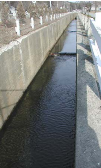
Long section of fishway
