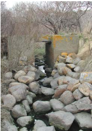
Old control structure at head of Salt Pond
