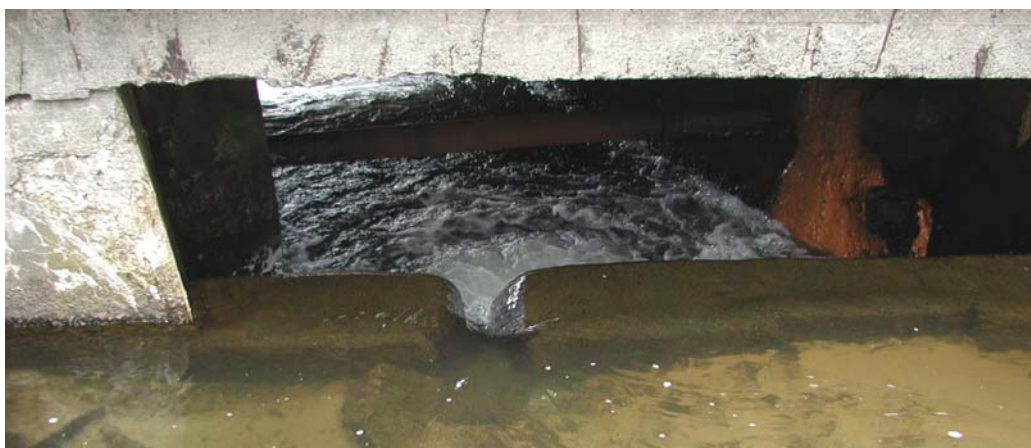
Water Street Dam (the notch in center is considered the fishway)
