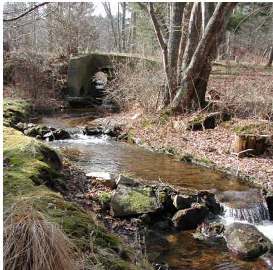
Stream baffles downstream of Brook Street culvert
