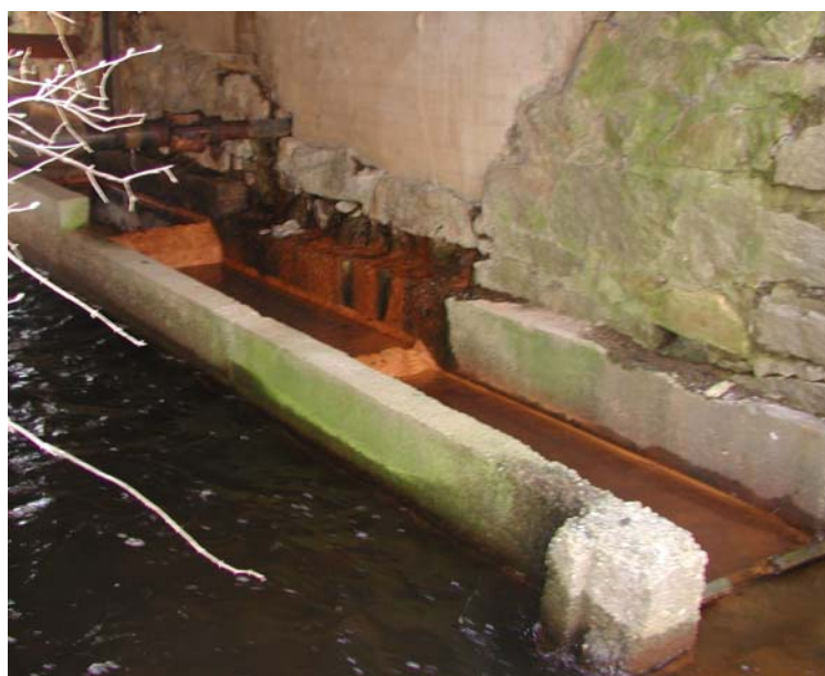
Russell Mill Pond fishway entrance (left) and fishway (right)
