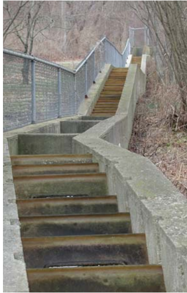
Mid-section of Newfield St. Denil fishway
