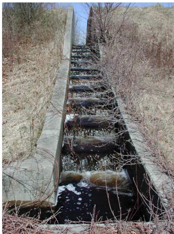
Upper section of fishway
