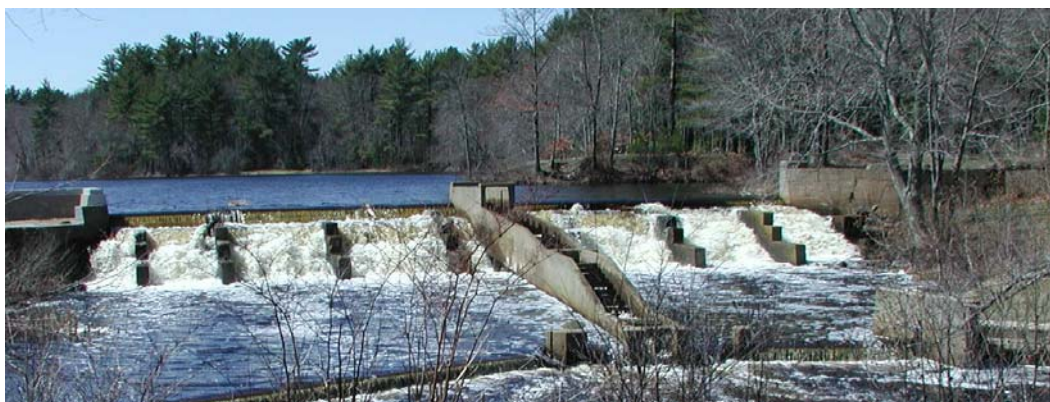
Elm Street Dam (fishway is in center of structure)
