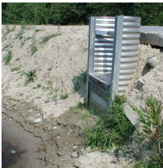
Bog sluice at North Hill Marsh (left) and outlet (right)
