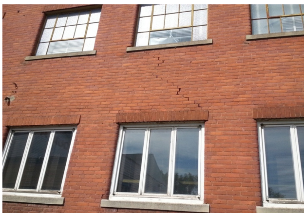
Figure 2-9. Cracks in masonry on east elevation of SHELd office building; photo from 2014 facility assessment by Reinhardt Associates.
