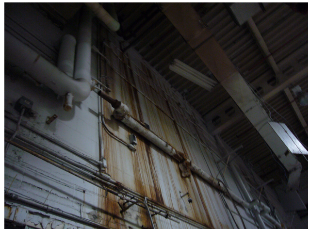
Figure 2-8. Evidence of roof leaks; pipes with potential asbestos insulation in Mill #6.
