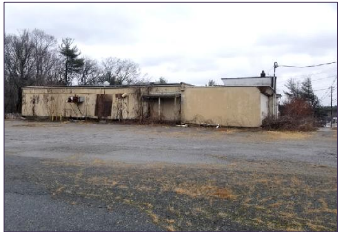
An underutilized commercial building on Rte. 9.
