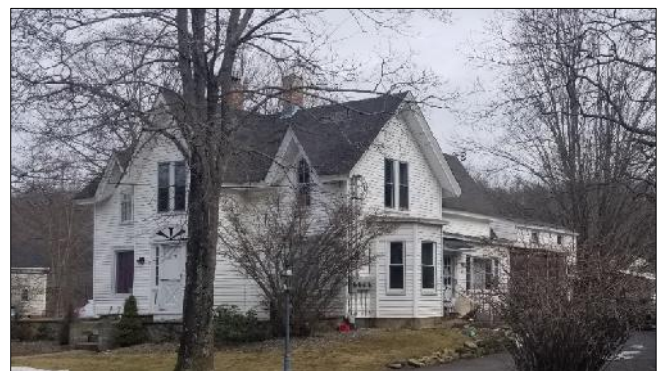
Small multi-family houses consistent with the New England architectural style could and currently do “fit in” in Southborough. The requirement for single-family homes limits the potential of the MRD regulations.
