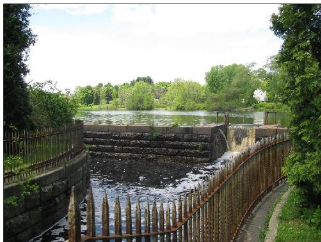
Deerfoot Road Aqueduct.
