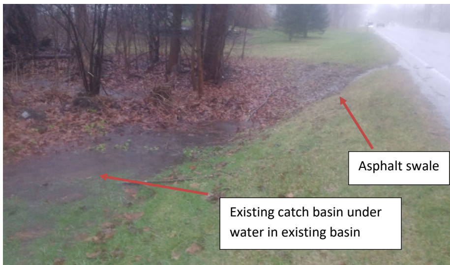
Photos C-8: Looking west along West Street shows existing basin (left) and eroded drainage channel which has formed off flowing off the driveway next to outfall pipe on property of 1161 West Street
