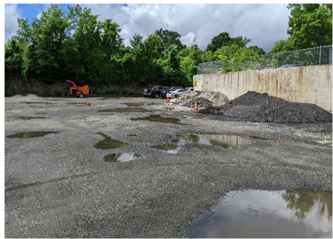
Photos C-1: DPW site, West Housatonic Street, Pittsfield. Upper photo shows the front parking lot where existing stormwater infrastructure could not be located. Bottom photo of parking lot entrance where asphalt is eroding and spalling.
