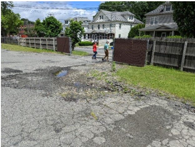
Photos C-1: DPW site, West Housatonic Street, Pittsfield. Upper photo shows the front parking lot where existing stormwater infrastructure could not be located. Bottom photo of parking lot entrance where asphalt is eroding and spalling.
