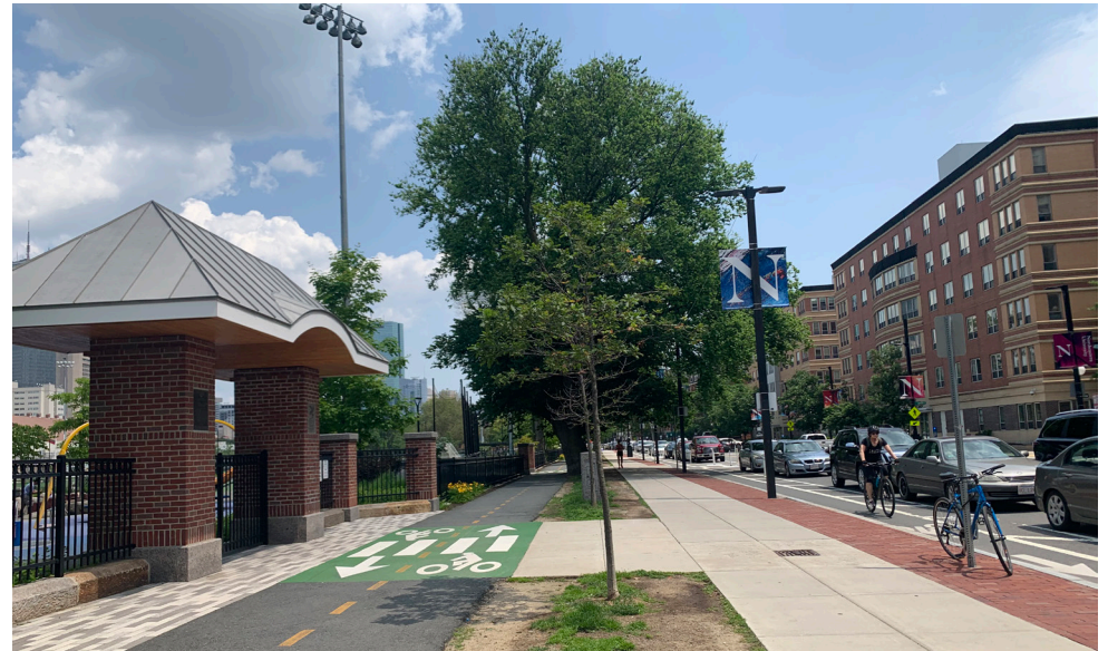
The Northeastern area includes a raised two-way bike lane and wide sidewalk area, and one-way protected bike lanes in the road
