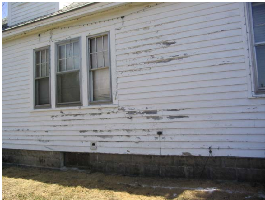
705-2B Family Development, 2 Babb Road Building Exterior – Paint Peeling on Side of House
