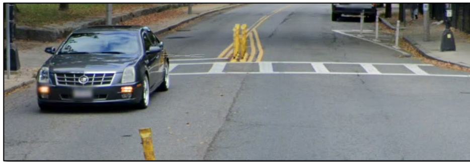
Figure 2.18: Centerline or corner hardening, Boston, MA
