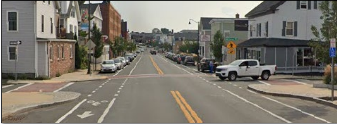
Figure 2.19: Intersection curb extensions, Beverly, MA
