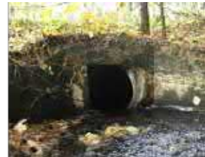
Inlet, Southbridge Rd (trib to Cady Brk)
