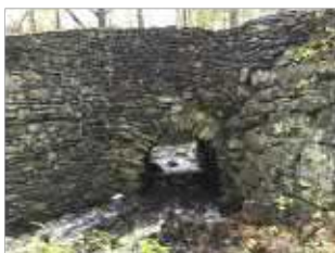
Inlet, Jones Rd
