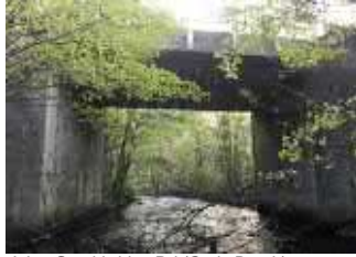
Inlet, Southbridge Rd (Cady Brook)
