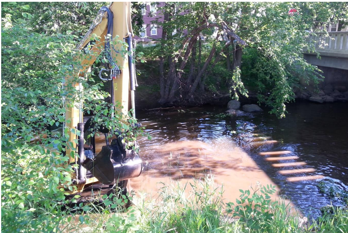
Random boulder cluster installation 50% Complete
