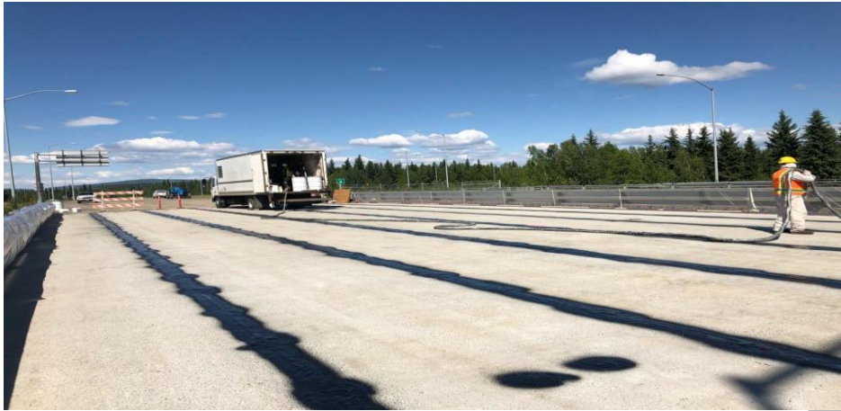
Figure 1 MagnoMembrane Filled Girder Joints
