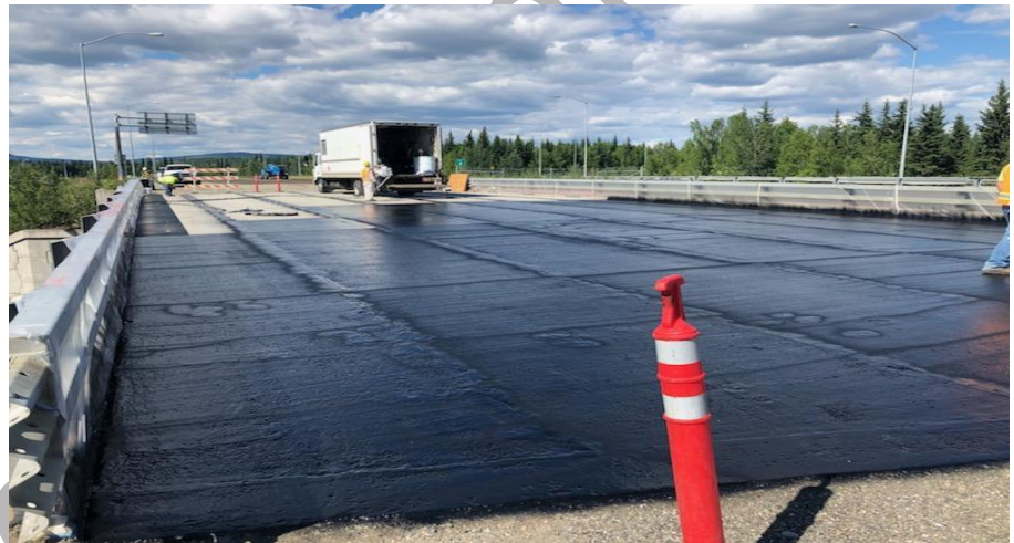
Figure 2 MagnoMembrane Base Coat without aggregate
