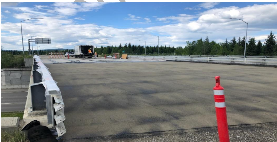
Figure 3 MagnoMembrane Top Coat with aggregate
