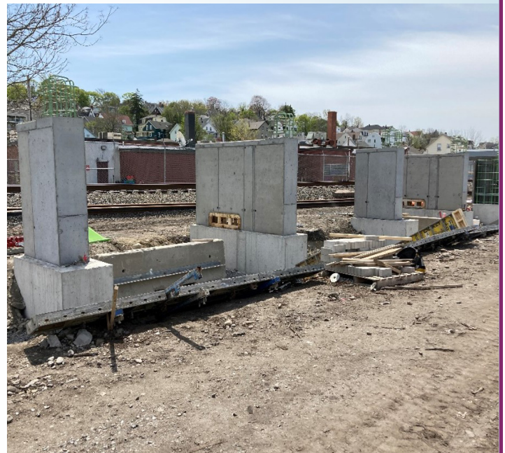
Platform support foundations at Fall River Station
