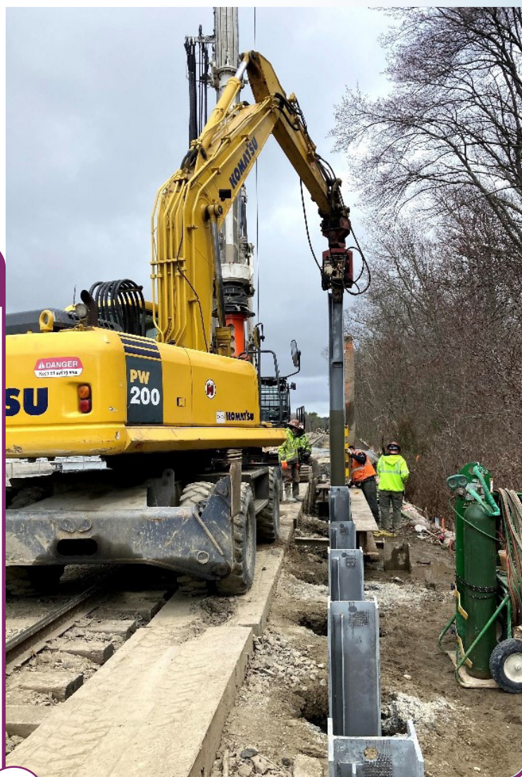
Installing soldier piles along the Fall River Secondary
