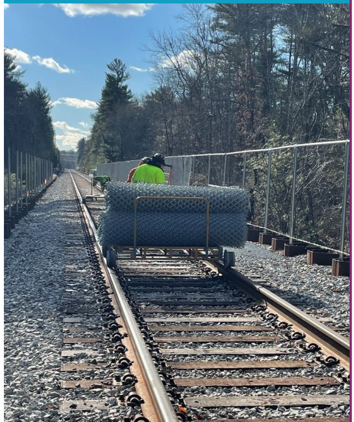
View of ongoing chain link fence operation
