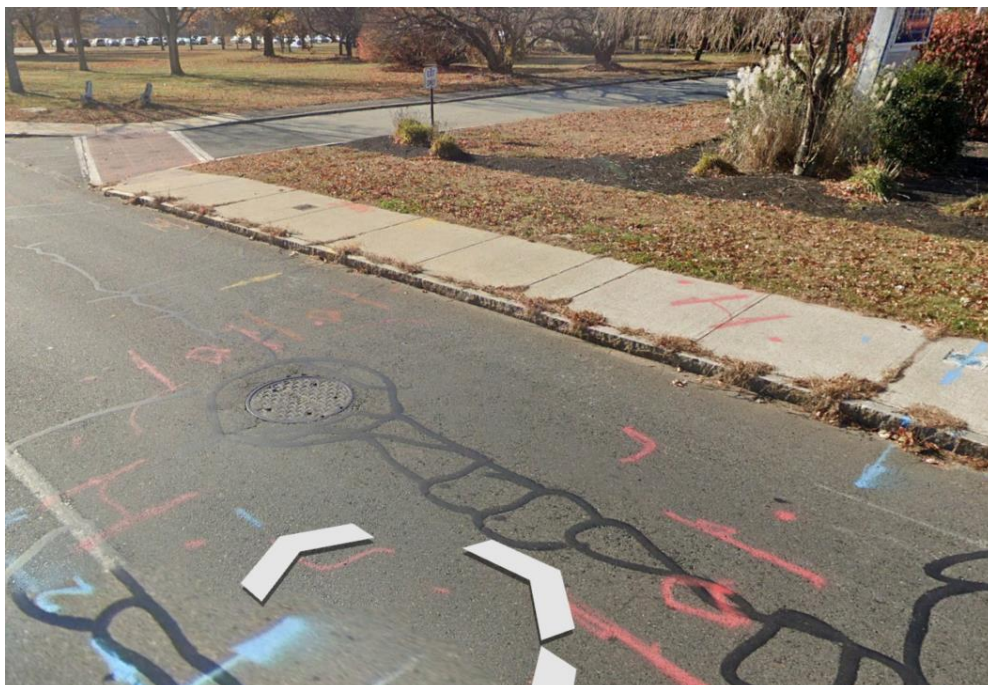
Eversource MH with electric pavement markings (source: Google Street View)
