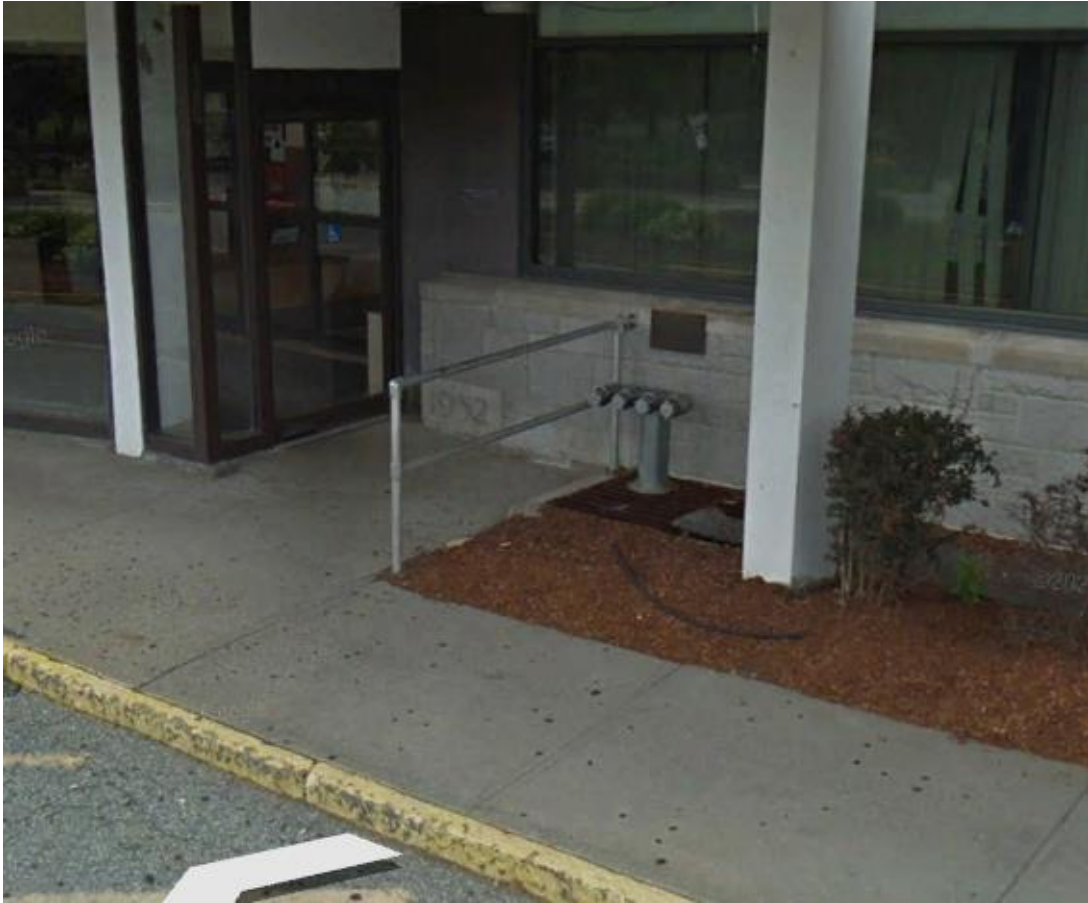
Fire connections at front of existing building (source: Google Street View)
