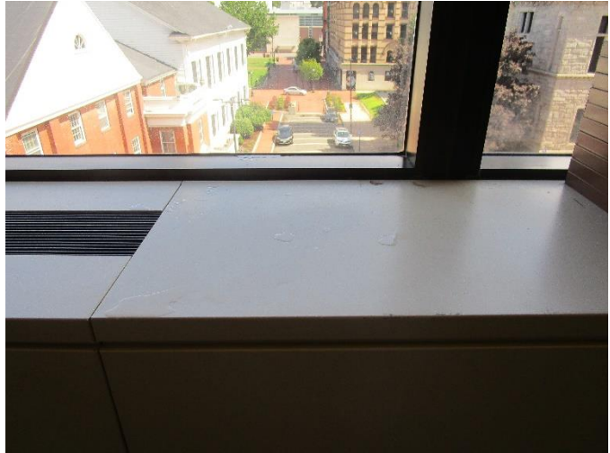
Photo 3: Water infiltration onto unit ventilator after rainstorm.
