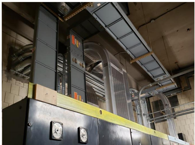
Photo 2: Above the original switchboard, which provides a junction for the old and new bus ducts.
