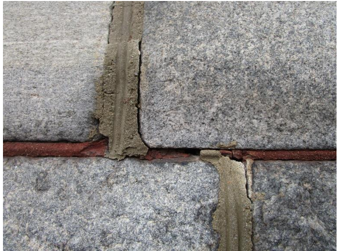
Photo 7: Example of grey and terracotta colored mortar in granite of Juvenile Court.
