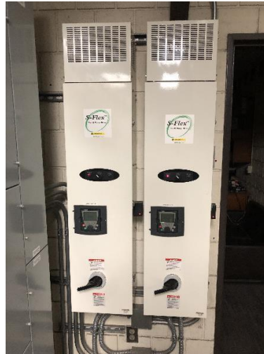
Photo 3: Cooling Tower Fan 1 & 2 Variable Frequency Drives (VFDs).
