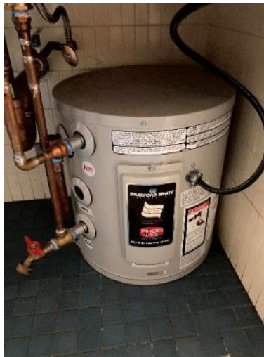
Photo 3: Bradford White LE11OU3-1NAL 10-Gal Electric Water Heater.
