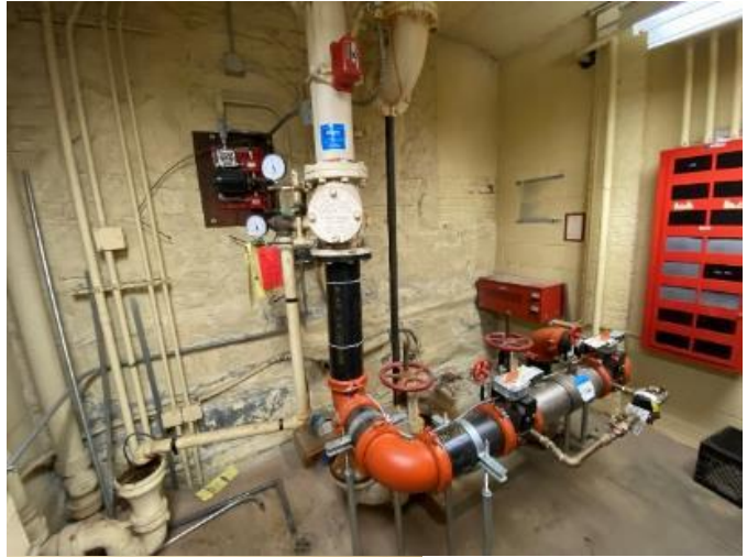
Photo 1: 6" Fire Service With 6" Wet Alarm Valve.
