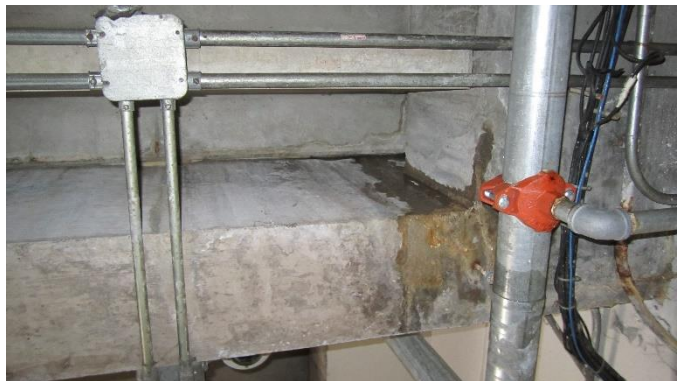
Photo 11: Water Infiltration at below grade parking.
