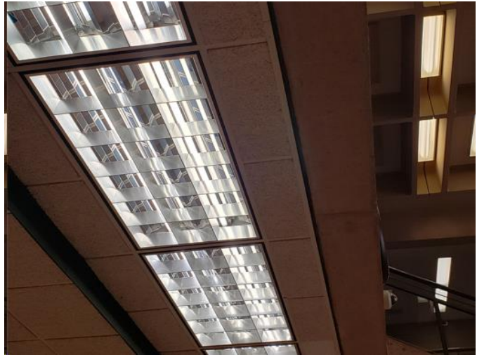
Photo 6: Light fixtures retrofitted with new LED lamps.
