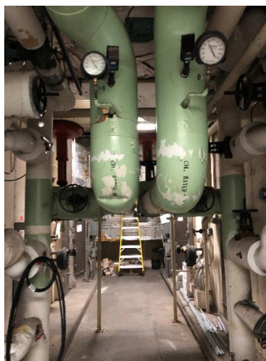
Photo 2: Chilled Water Piping Serving AC-3 & AC-4.
