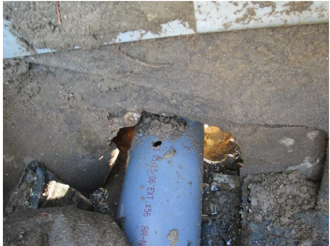
Photo 13: No waterproofing at below grade scuppers
