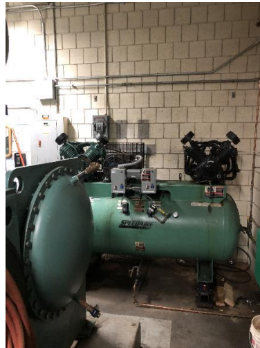
Photo 4: Air Compressor Serving Pneumatic Controls.
