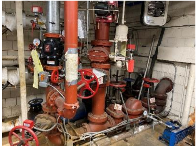
Photo 1: 8" Fire Service With 6" Wet Alarm And 6" Dry Valves.
