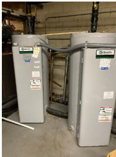
Photo 2: (2) A.O. Smith DRE-80 100 Electric Water Heaters.
