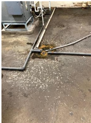
Photo 5: Mechanical Floor Drain Overflow.
