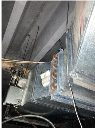
Photo 15: Typical Reheat Coil (Smaller than Upstream/Downstream Ductwork).
