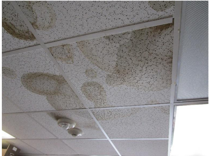
Photo 6: Damaged ceiling in Room 301, which is the room below the tower.
