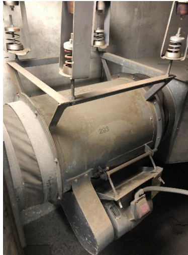
Photo 24: Supply Fan Believed to Serve Smoke Control System.
