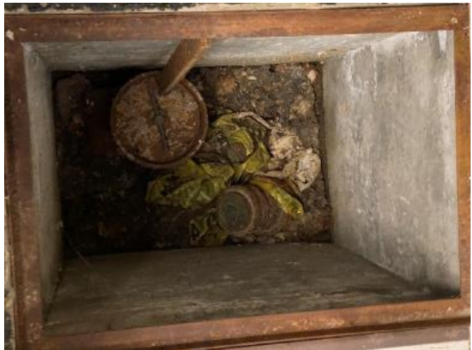
Photo 4: Failed Waste Main Check Valve.
