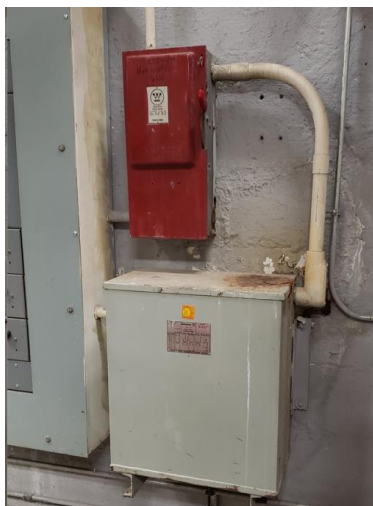
Photo 2: Rusted transformer enclosure under leaky spot in mech room.
