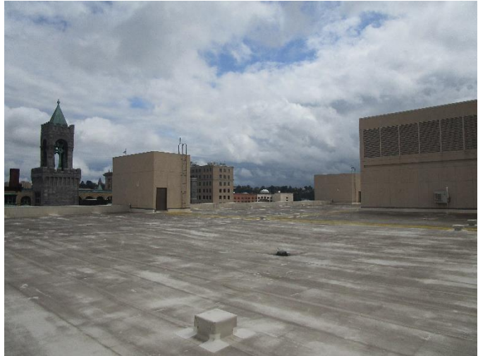
Photo 10: Thermoplastic roof with stair and mechanical penthouses.
