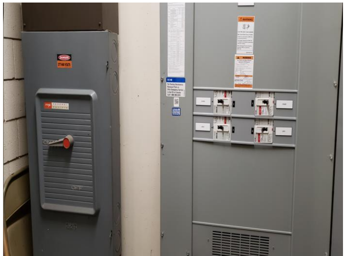
Photo 4: Original Federal Pacific Disconnect Switch and Newer Distribution Panel.
