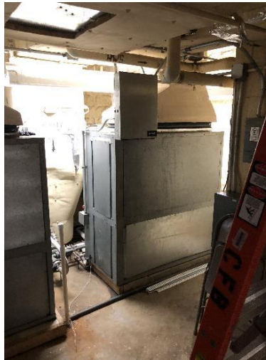
Photo 1: Basement Mech Room Typical Vertical Air Handling Unit.
