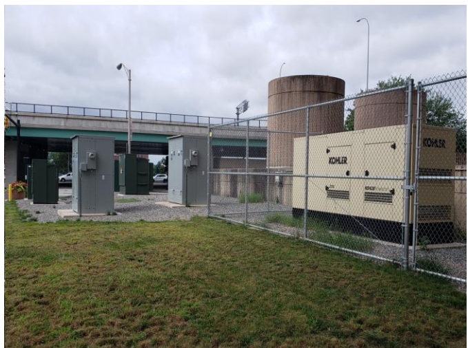
Photo 5: 200KVA Generator and exterior pad-mounted utility transformers for both buildings.
