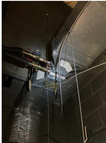
Photo 16: Typical Reheat Coil (Smaller than Upstream/Downstream Ductwork).
