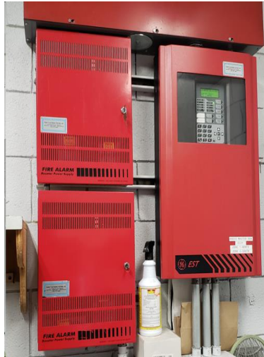
Photo 3: Fire Alarm Radio Master Box and Power Supplies by GE.
