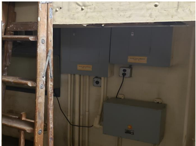
Photo 1: Ductwork intruding on clear working space of power panels.
