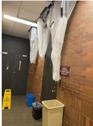
Photo 21: AC-1 Failed Drain Pan – Leaking Above Hallway.
