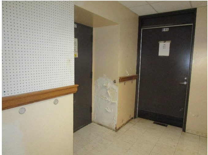
Photo 3: Moisture damaged walls in basement. Note vents added in wall assembly as attempted repair to reduce moisture buildup and peeling paint.
