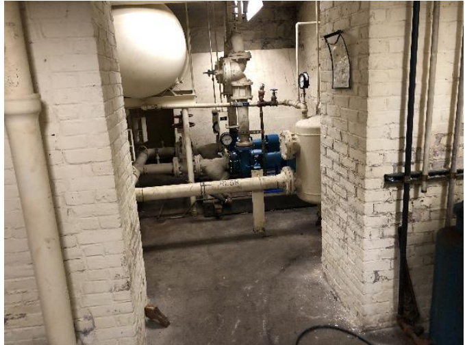
Photo 6: Base-Mounted Pumps, Expansion Tank, Air Separator, etc.
