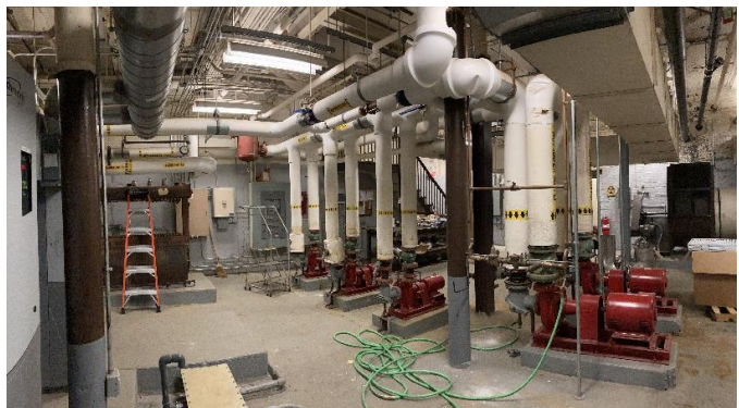
Photo 23: Typical Base-Mounted Hot Water Pumps.
