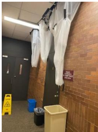
Hall of Justice – AC-1 Failed Drain Pan – Leaking Above Hallway
