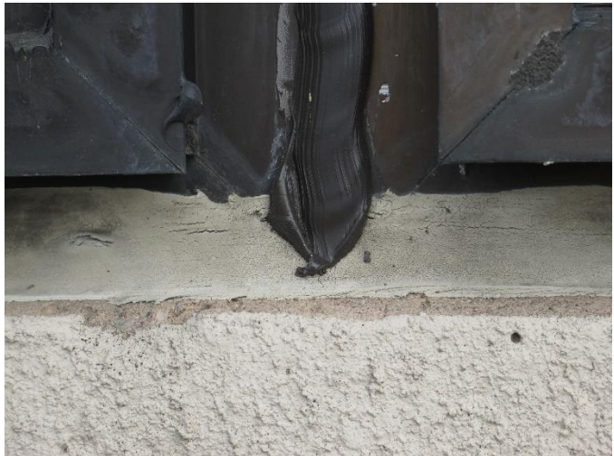
Photo 9: Deteriorated sealant at window.
