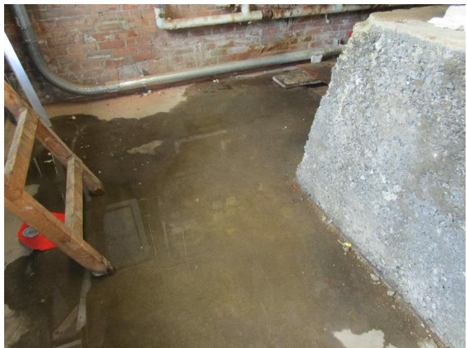
Photo 4: Water infiltration in basement after rainstorm.
