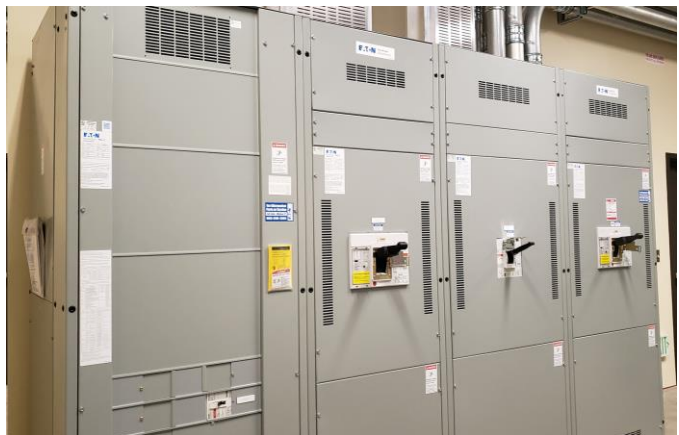
Photo 1: Existing 208/120V Switchboard in Main Electrical Room.
