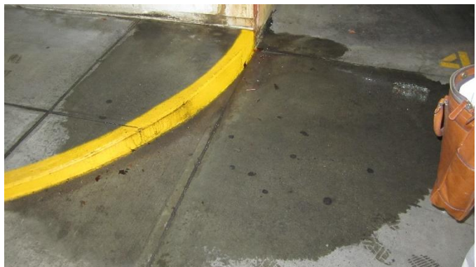
Photo 12: Evidence of water infiltration at parking garage.
