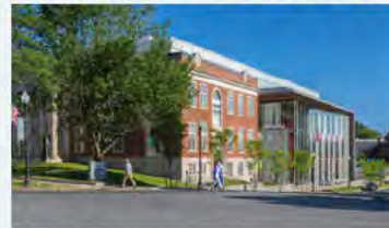
Franklin County Justice Center Greenfield, MA
