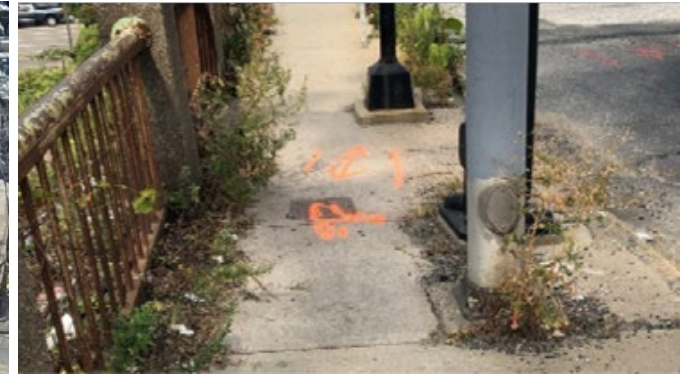
Insufficient clearance around equipment
