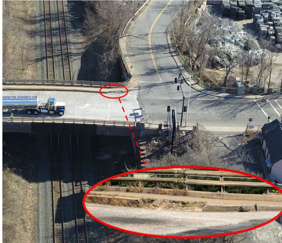
Tight turning radius at Albany Street; damage at the curb
