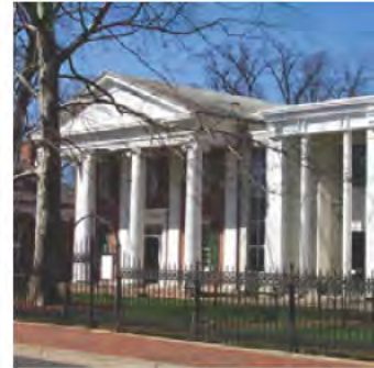
Loudoun County Courts Complex Leesburg, VA
