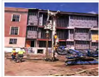
Mini-Pile drilling rig installing first drilled mini pile
