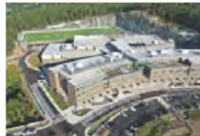
City of Waltham, High School WALTHAM, MA
