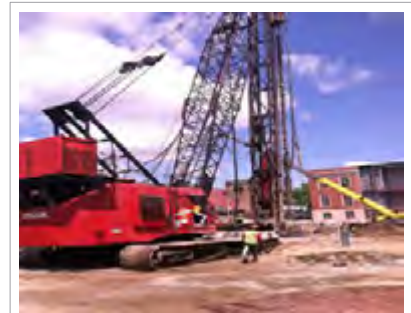
Pile Driving Crane with Pre-Auger attachment
