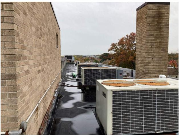
Figure 9: Rooftop Air Cooled Condensing Units at Ellison
