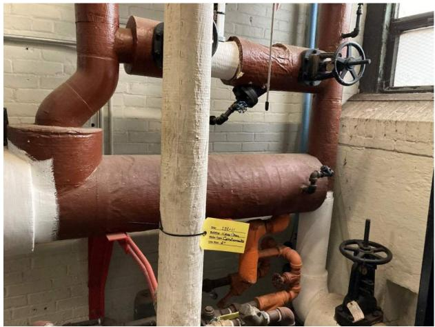
Figure 10: Incoming Steam service and Heat Exchanger at Horace Mann
