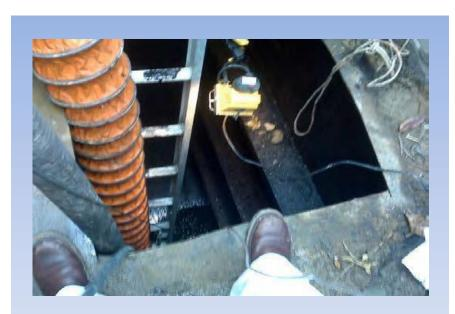
Ventilation hoses provide air and exhaust toxic vapors during permit required confined space entry.
