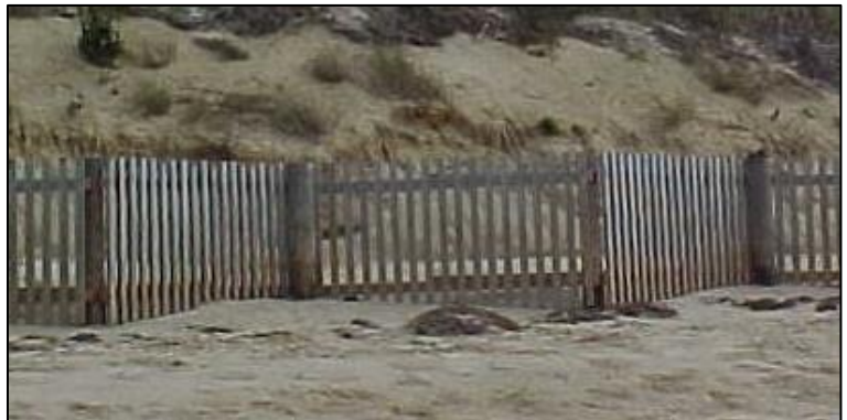
This sturdy drift fencing is constructed in a zigzag pattern parallel to the shoreline with 2x3-inch vertical and horizontal cross-members attached to 6- to 8-inch posts. As described above, this type of fencing is not recommended because of its adverse impacts. (Photo: CZM)
