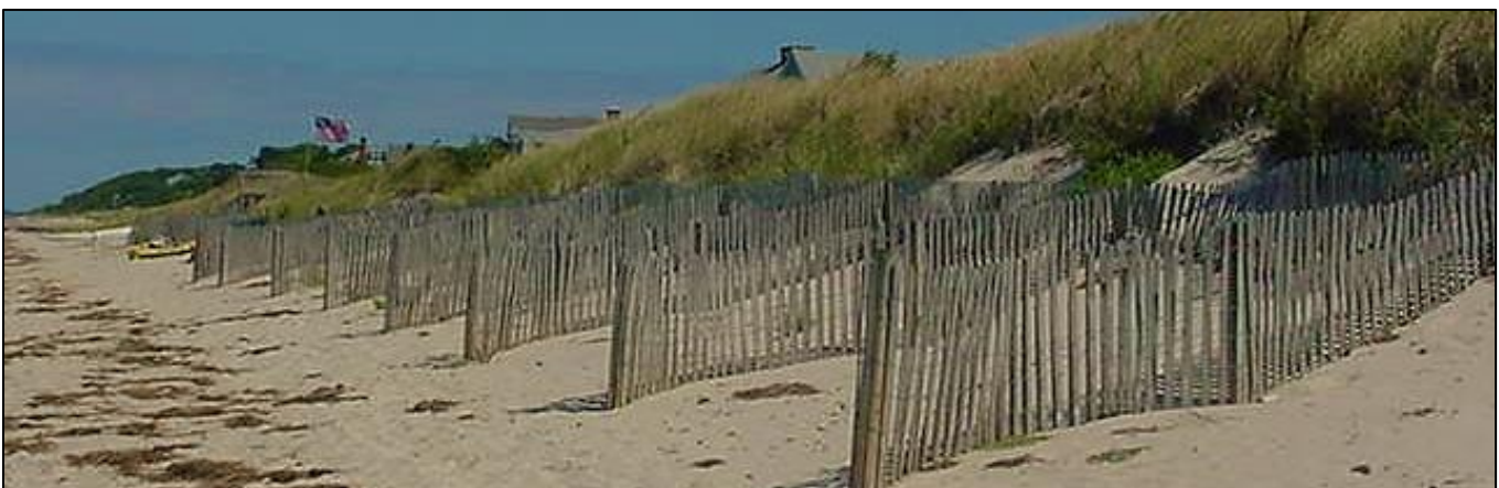
Sand fencing was installed along the base of and perpendicular to this eroded dune to trap windblown sand and help rebuild the dune. (Photo: CZM)
