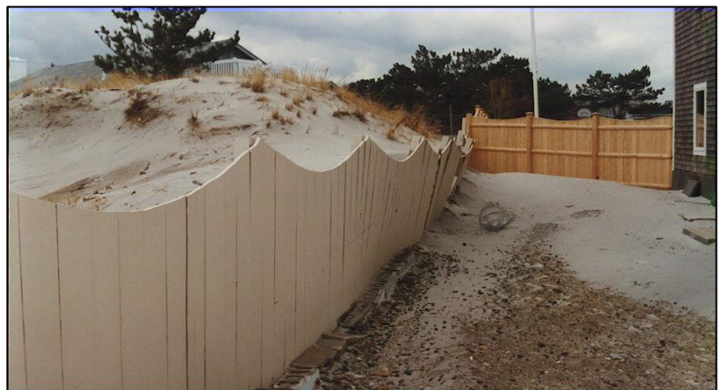
A solid fence prevents the natural movement of this dune. (Photo: CZM)
