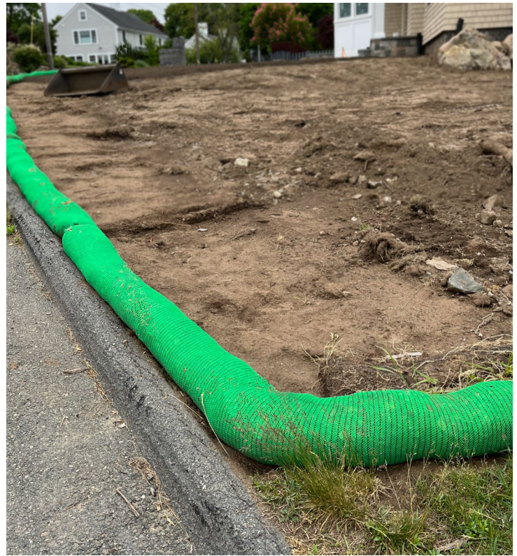
Compost filter socks can be placed down slope from exposed soils to prevent muddy water from flowing offsite and into roads, adjacent yards, or wetland resource areas.
