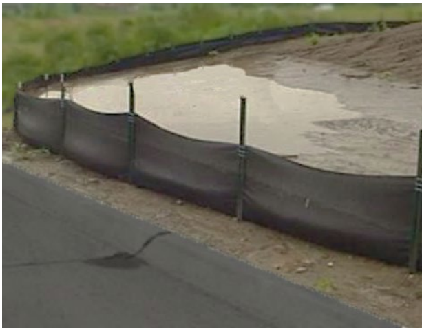
Silt fence surrounding exposed soils
