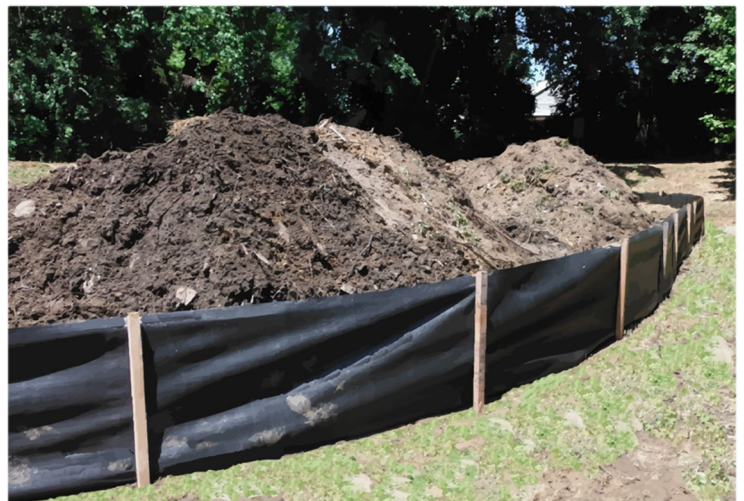
A silt fence installed around a pile of topsoil helps prevent sediments from being washed into storm drains and waterbodies when it rains.
