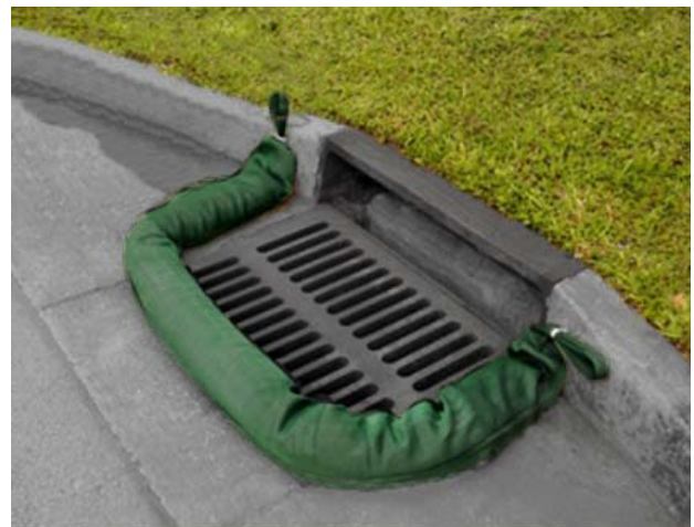
Compost filter sock surrounding a storm drain
