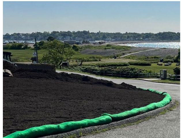
Compost filter sock surrounding exposed soils
