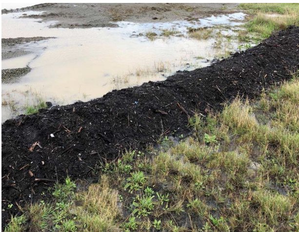
Compost filter berm to slow and divert water
