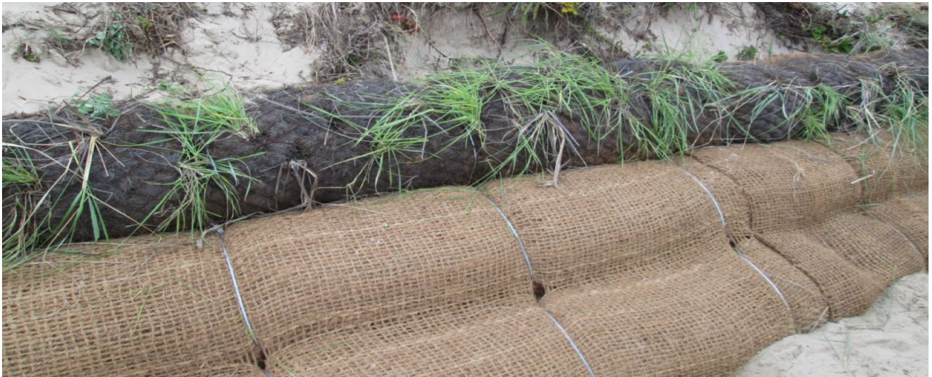
Top row: An erosion-control blanket was installed next to a cove and planted with salt marsh grasses. The blanket provides a stable medium for the plants to grow while preventing erosion of exposed sediments. Bottom row: Coir rolls were installed along a coastal bank, one of which has been planted with vegetation prior to installation.
