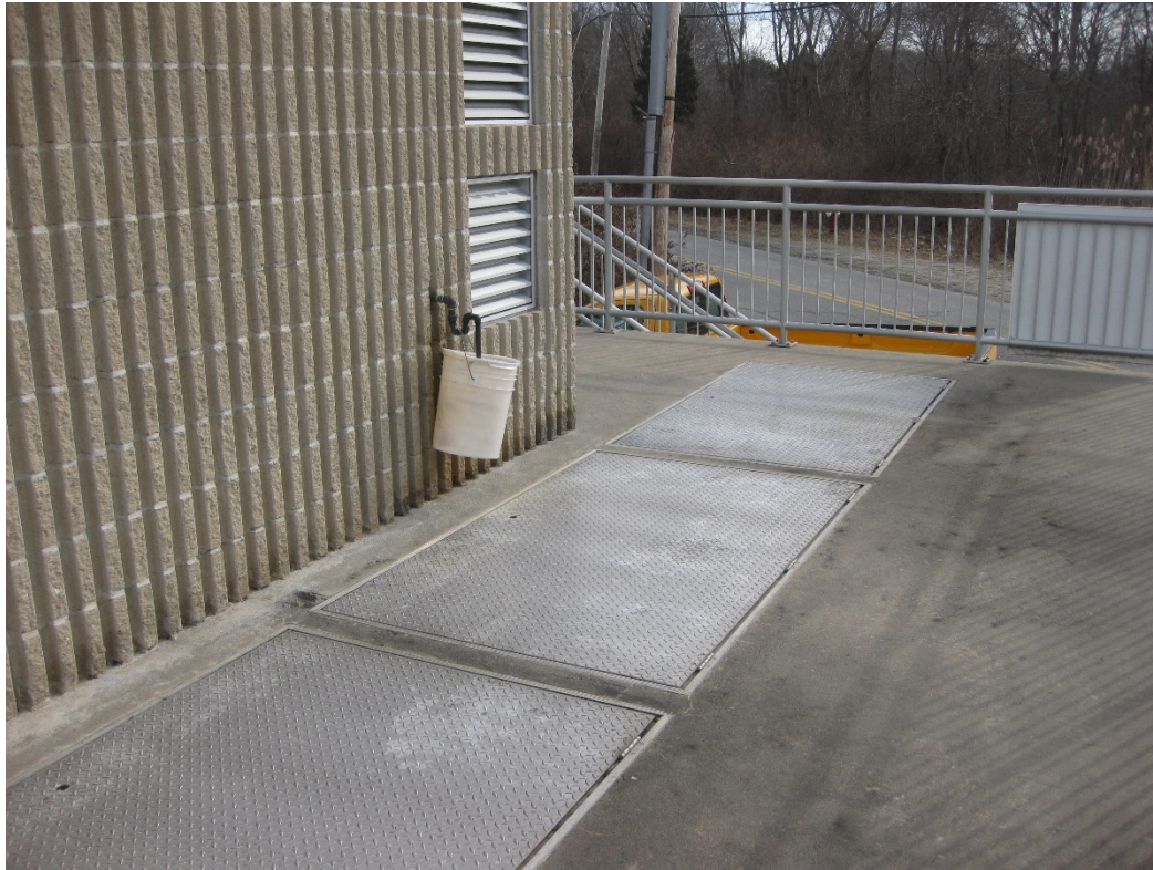
Photo #3 – Equipment hatches at main slab exterior
