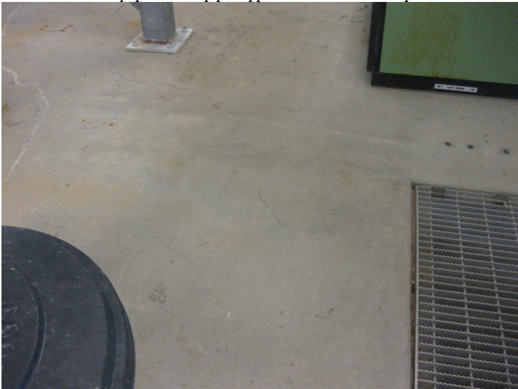
Photo #12 – Cracks at the slab on grade
