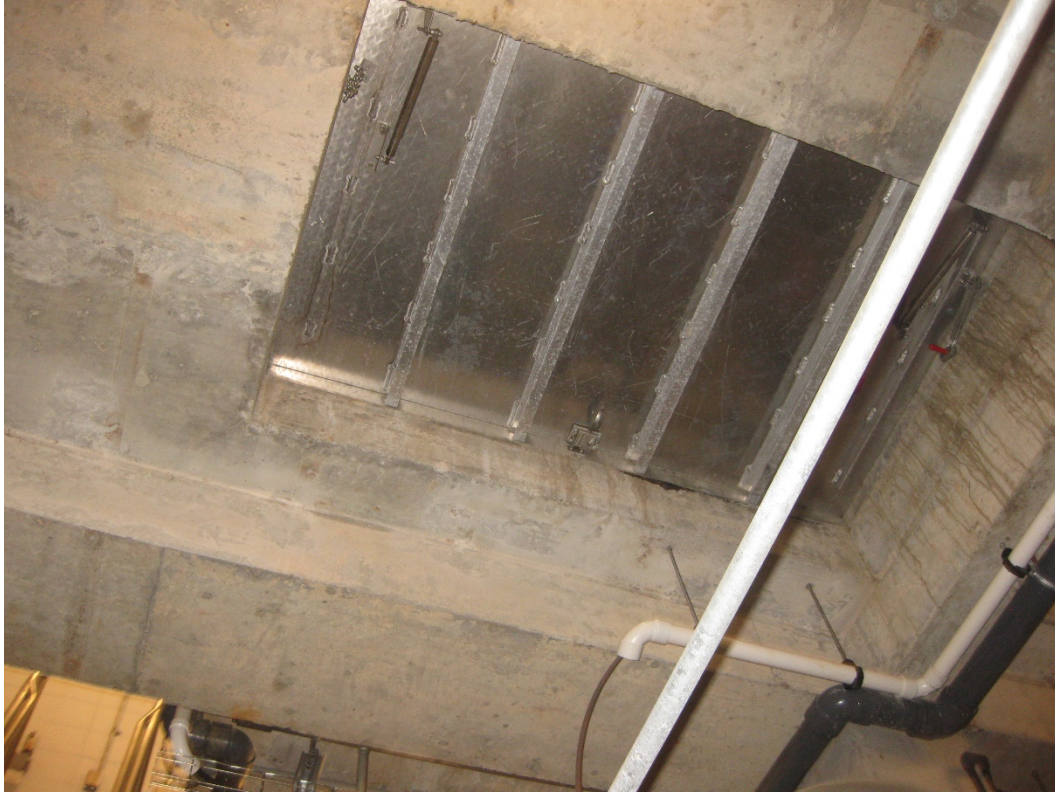
Photo #7 – Water stains at underside of equipment hatches
