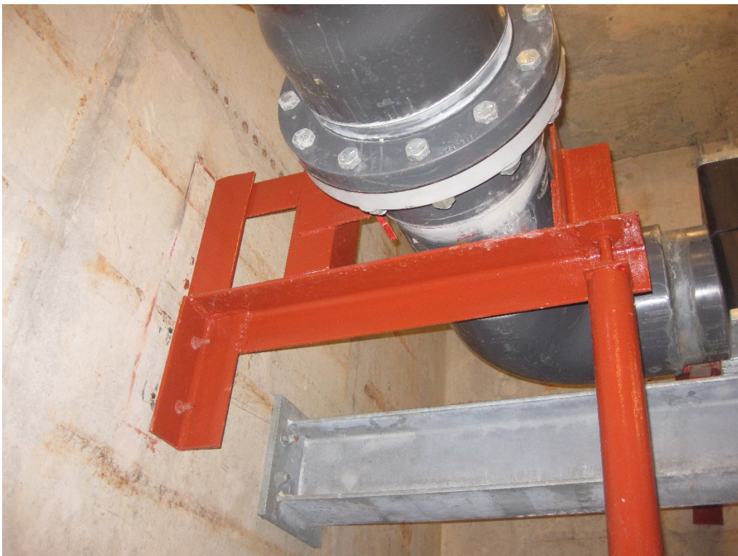
Photo #10 – Painted steel pipe supports
