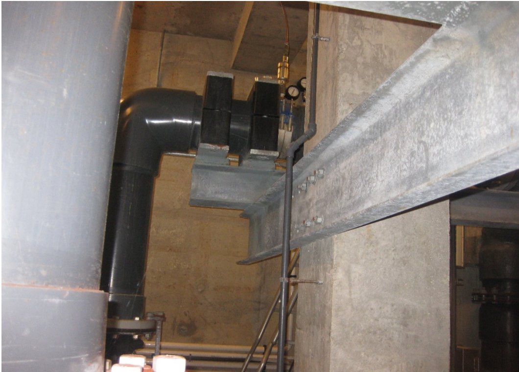
Photo #9 – Galvanized steel pipe supports
