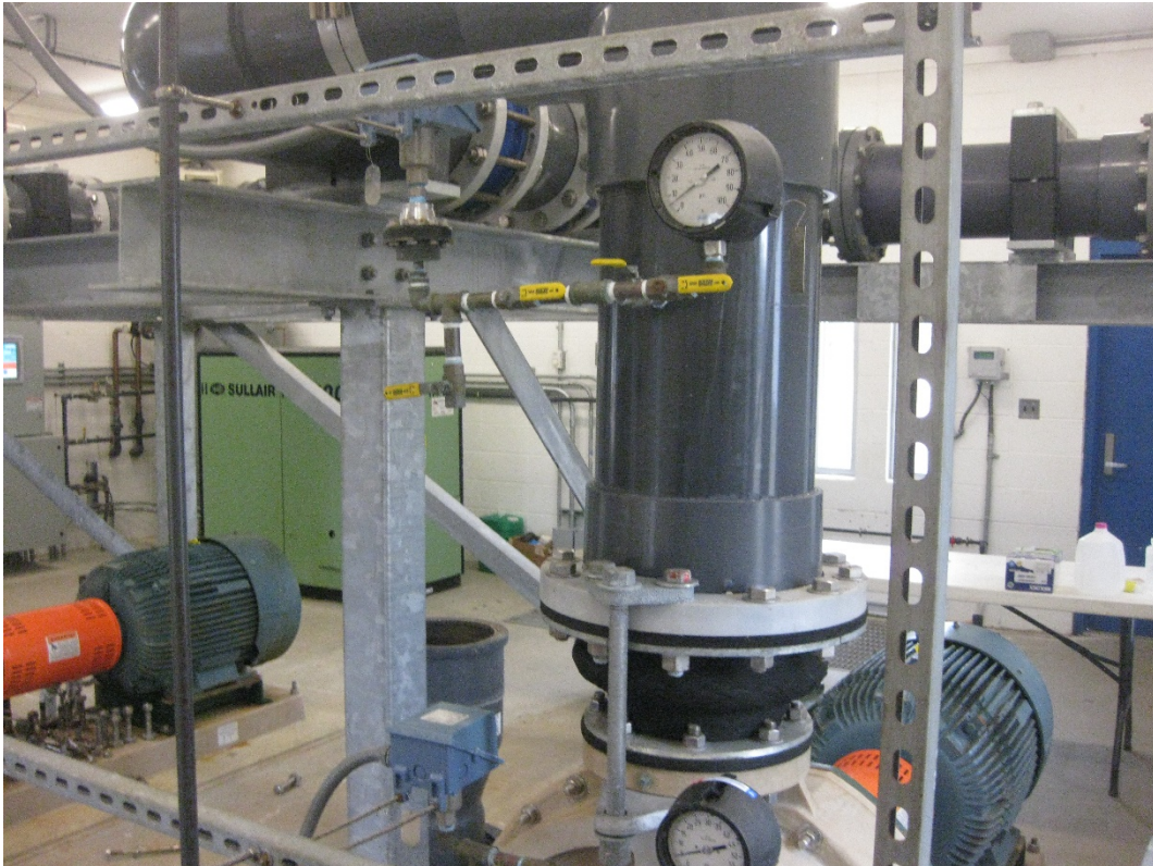
Photo #11 – Equipment and pipe supports at Raw Water Pump Station
