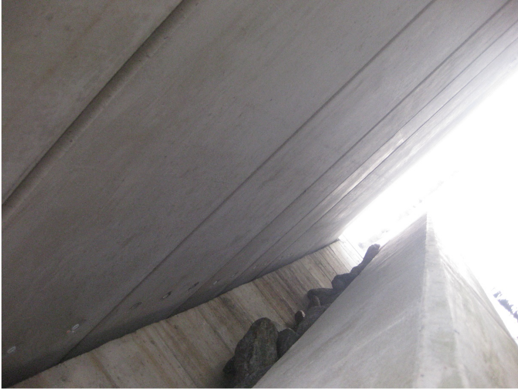
Photo #15 – Signs of water infiltration at abutment
