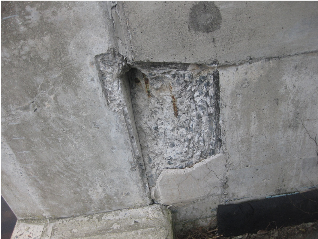
Photo #14 – Spalling at bridge abutment
