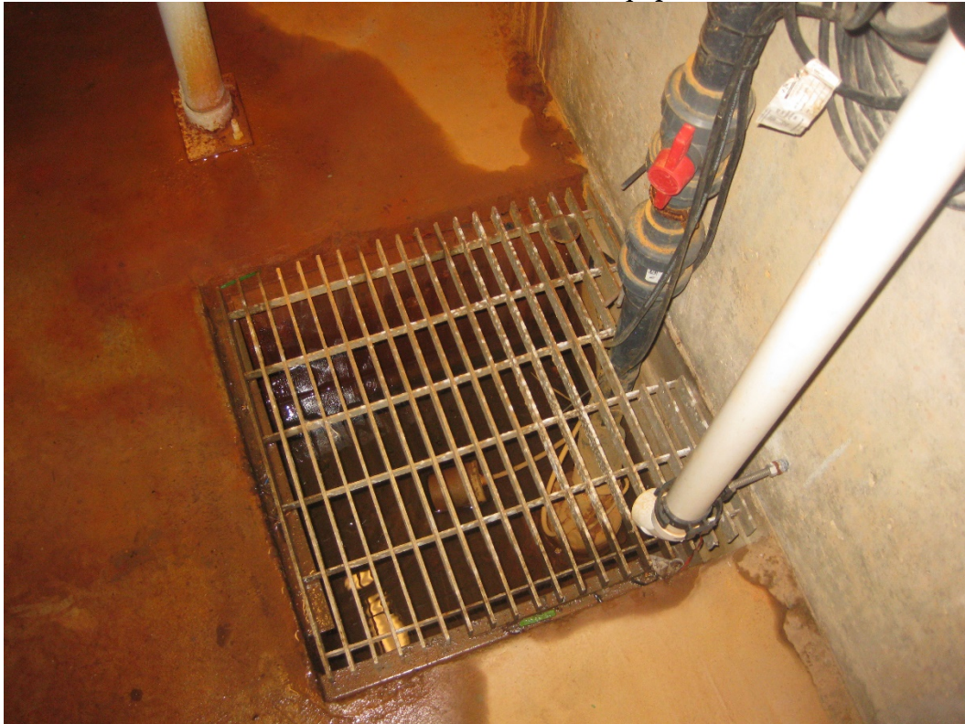
Photo #8 – Sump pit in basement level
