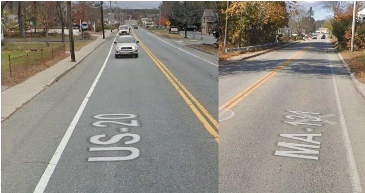
Pictures above show sidewalks in right of way that are proposed to be treated.
