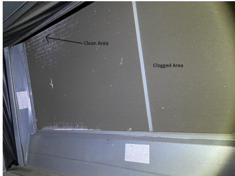
Photo 2 – Typical Clogged Condenser Coil
