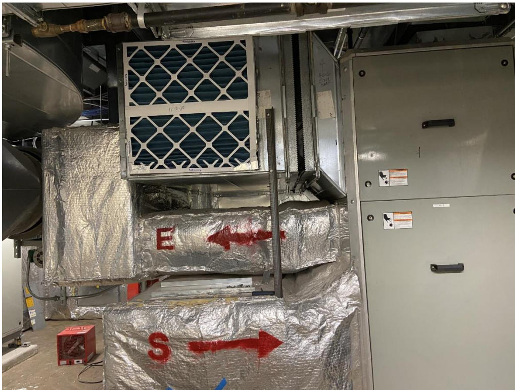
Photo 1 - AC-7 (right) with Return Air Filter in Mechanical Room
