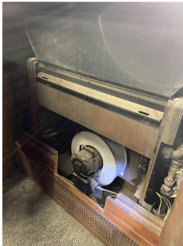
Photo 3 – Courtroom 1006 Unit Ventilator
