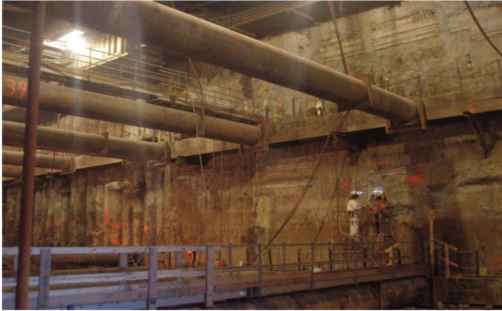
Figure 6: Slurry Walls as Permanent Support, Bottom-Up Construction, Second Avenue Subway Phase One (96 th Street Station)
