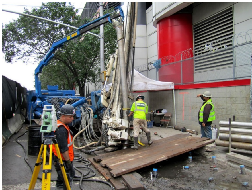
Figure 10: Ground Freezing from Surface, Extension of the NYCT No.7 Line Subway, New York, NY
