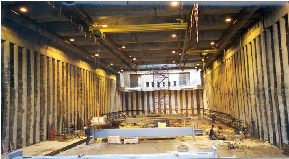
Figure 7: Secant Piles as Permanent Support, Top-Down Construction, Copenhagen Metro
