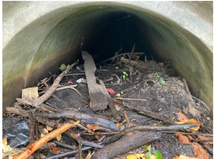
Looking South – Pond outlet partially blocked by debris
