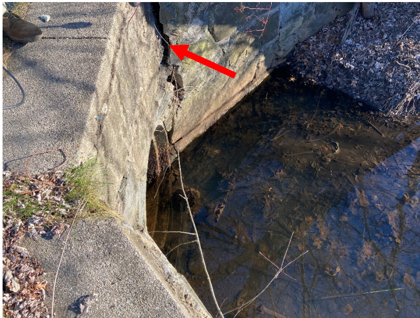
Two-inch crack in the headwall at the Main Street culvert inlet
