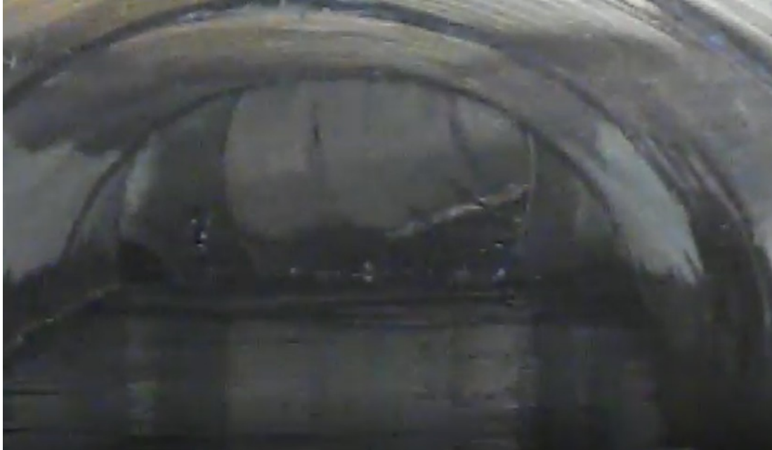
Main Street Culvert transitions from 36-inch RCP to a 38-inch X 57inch CMP
