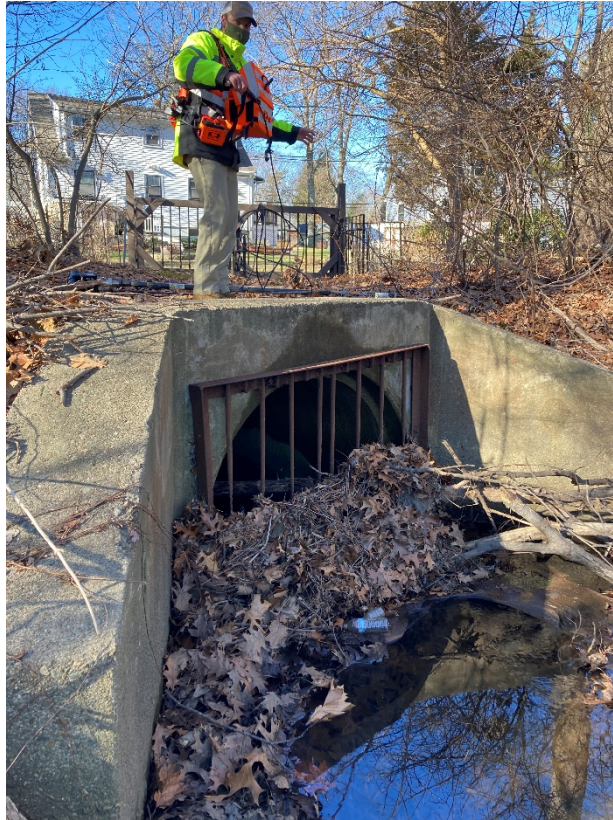
Debris blocking flow at the culvert inlet near Fuller Middle School
