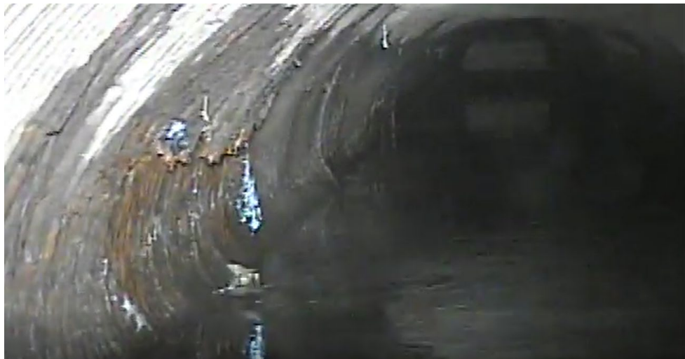
2-foot x 2-foot deteriorated metal pipe section. Active groundwater infiltration observed.
