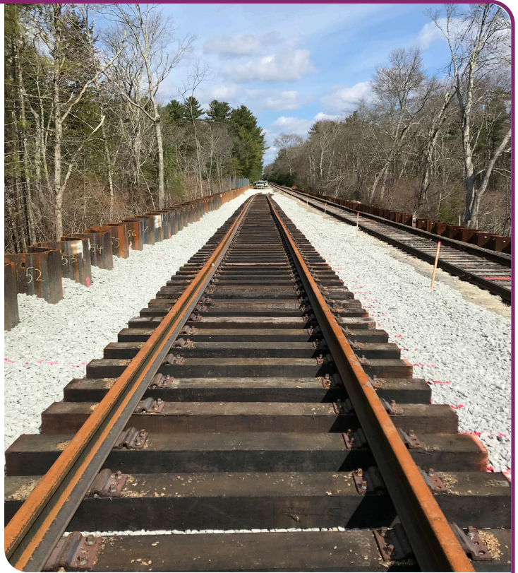
Completed segment of rail over a culvert.
