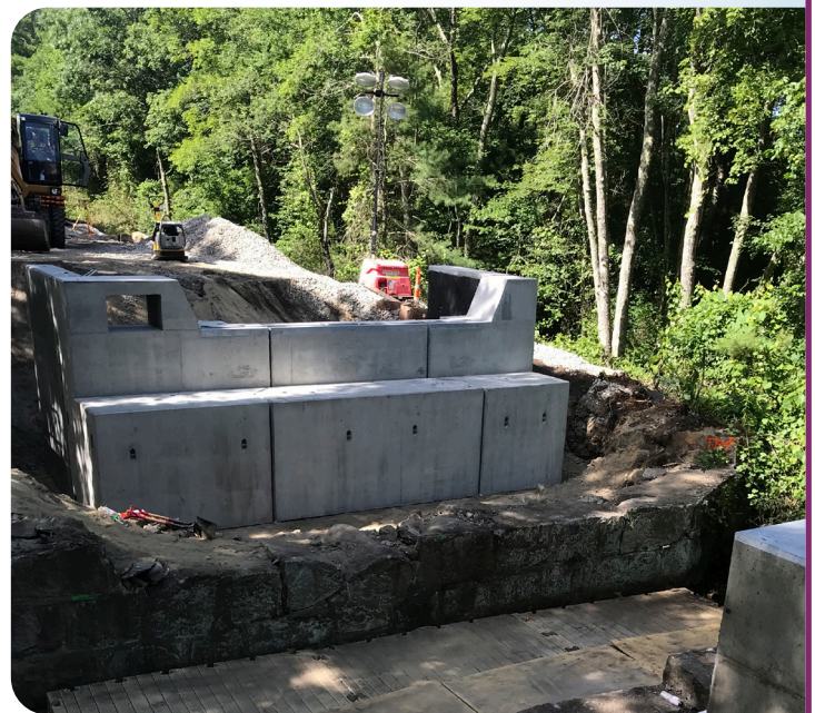
The abutment walls for the new Fall Brook Railroad Bridge in Freetown are installed (July 2020).
