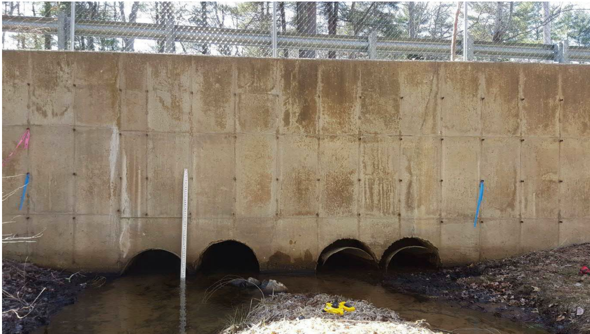
Figure 6. Bayberry Lane Culvert Complex
