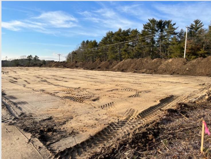
Subgrade materials graded, organics stockpiled and ready to be spread
