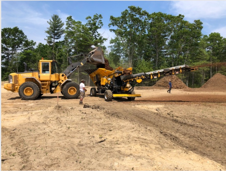
Spreading native wood chips after planting cover crop and prior to PV installation
