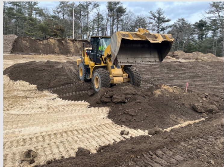
Re-spreading organics and after bog sand removal and subgrade prep
