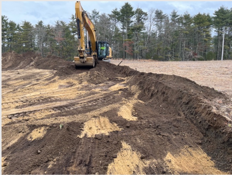
Stripping & stockpiling organic materials after clearing and prior to sand excavation
