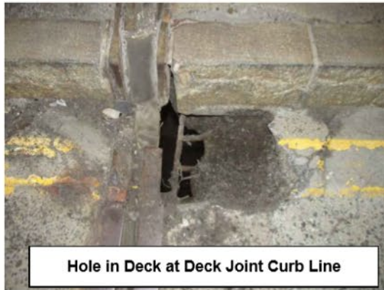
Corrosion of SIP Forms/Exposed Deck Rebar
