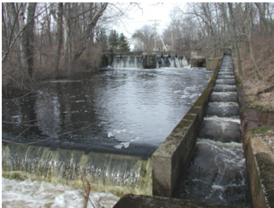
Fishway at High Street, with dam in background
