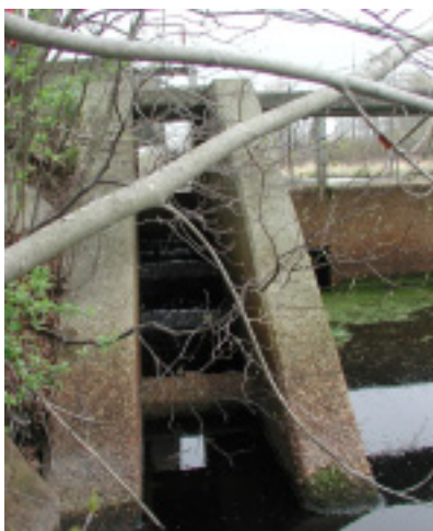
Fishway at Stump Brook Dam
