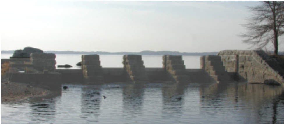
Assawompset Pond Dam (with Fishway along left edge of the dam)
