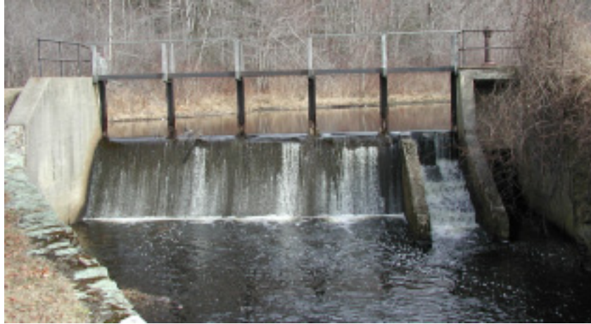
Forge Pond Dam, with fishway along right edge of the dam
